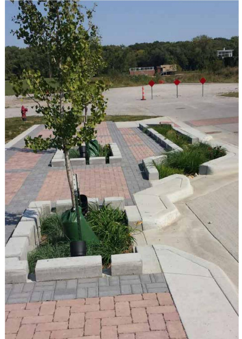
Figure 112: Stormwater planters intercept and filter road and sidewalk runoff during small storms, this example is at Iowa River Landing Place in Coralville. Also visible in the foreground is a permeable paver brick sidewalk.
