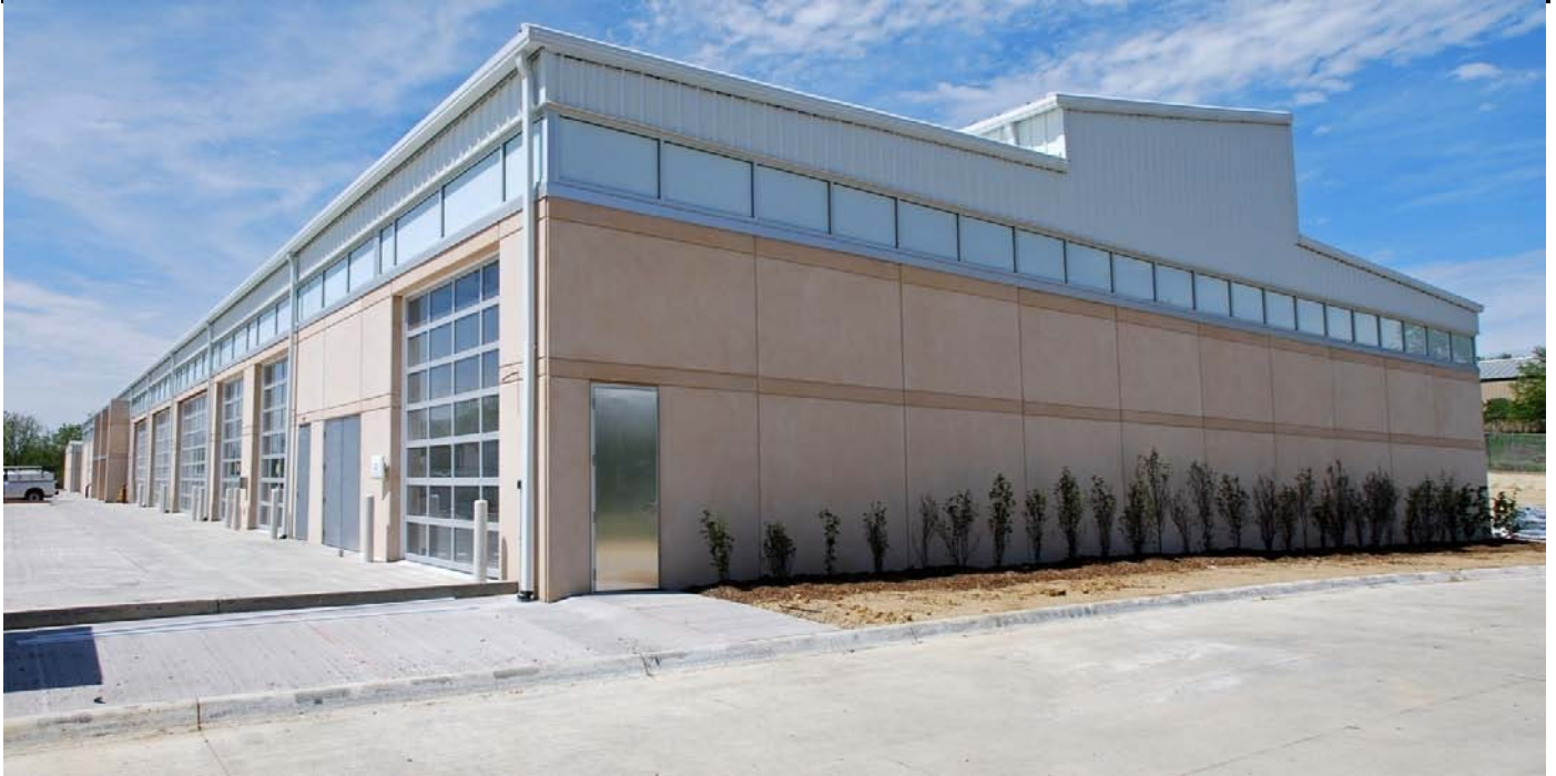
Parks, & Transit Maintenance Facility
